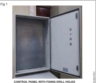
CONTROL PANEL WITH FIXING DRILL HOLES
