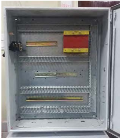
CONTROL PANEL WITH RACEWAYS/DIN RAILS
